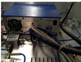
output selector box indicating missing power
