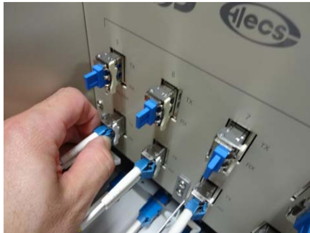
Figure 15: Pulling out the optical fiber
